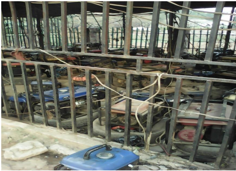
Figure 5. Power House with Indiscriminate Arrangement of Small Size Electric Power Generators in Wuse market [Source: Odaudu, 2021 in the Repository of the Federal University of Technology, Minna, Nigeria ( http://repository.futminna.edu.ng:8080/jspui/bitstream/123456789/12657/1/ODAUDU%2C%20Ugbede%20Sunday-%20PhD-SET-2015-665.pdf ); Retrieved on 06/04/2023].
