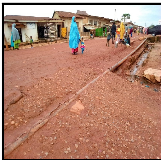
Figure 12: Blocked Water Pipe Filled with Sand Source: Author's Field Survey, 2018
