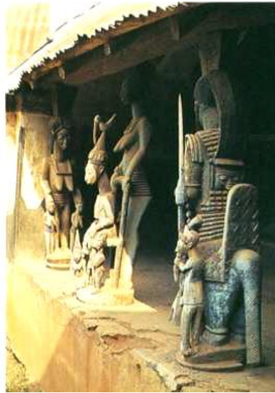
Figure 12: Sculptural Image Used as Structural Column in Traditional Yoruba Building.
